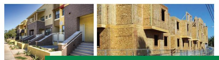
SIP panels come precut from the factory per your custom plans. SIPs can be ready for siding/roofing much faster than traditional framed construction and insulation.
