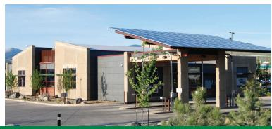
The high performance rigid insulation in the Premier SIPS walls and roof increase energy performance for the long term.
