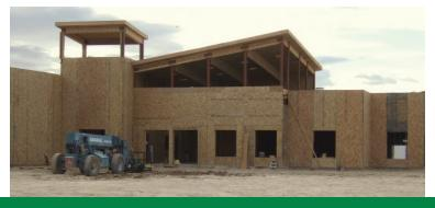
Prior to SIPs, contractor had allocated 12 men for the electrical installation, ended up needing only 3 and reduced their original bid by over \$950,000.
