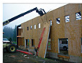
SIP construction has far fewer gaps than other framing methods.
