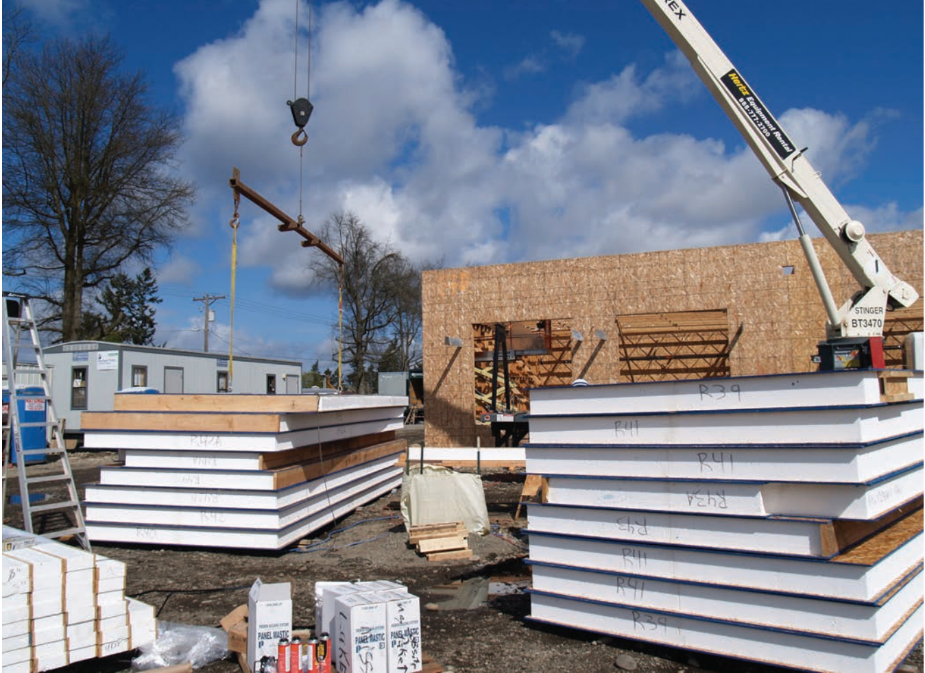
BUILDER STAGES SIPs at a jobsite for rapid installation.
