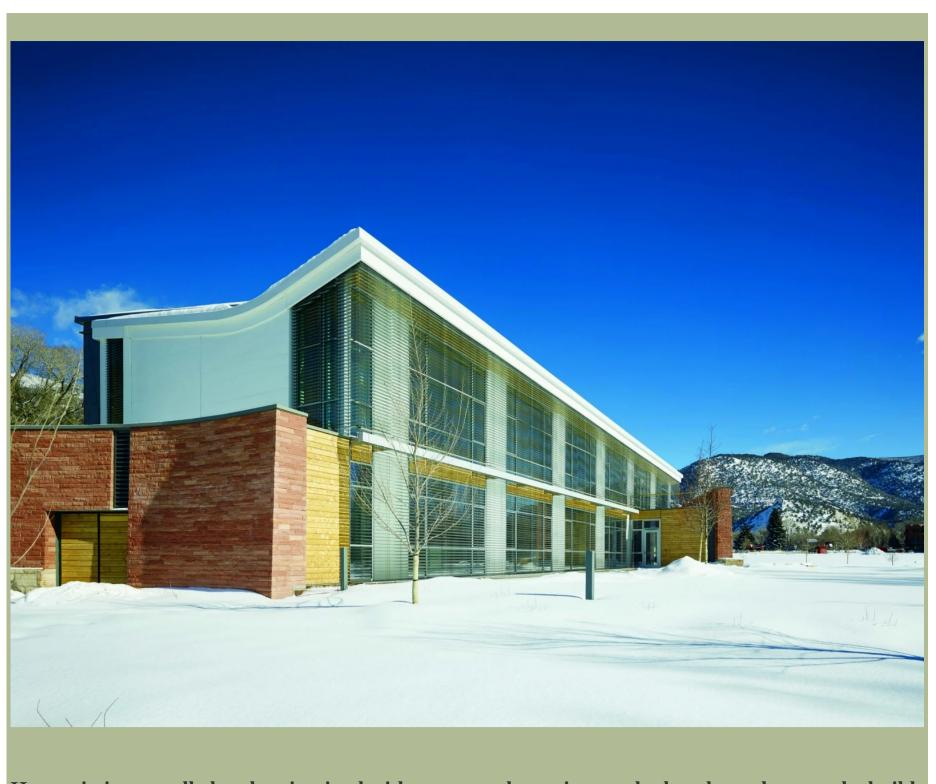
Heat gain is controlled and maintained with automated exterior sunshades, shown here on the building's south façade.
