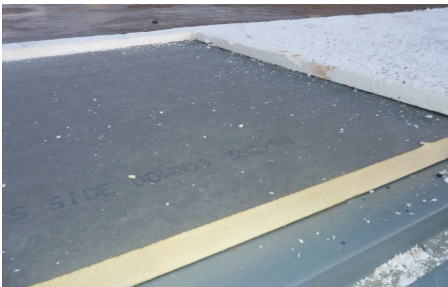
Figure 3. Existing roof being removed
