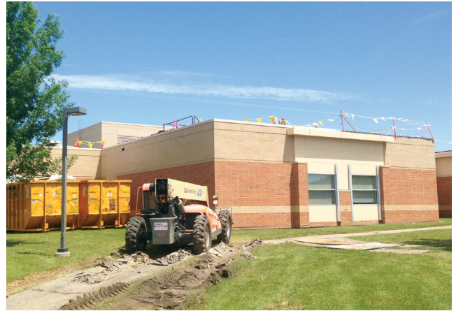
Figure 2. Roof replacement in progress
